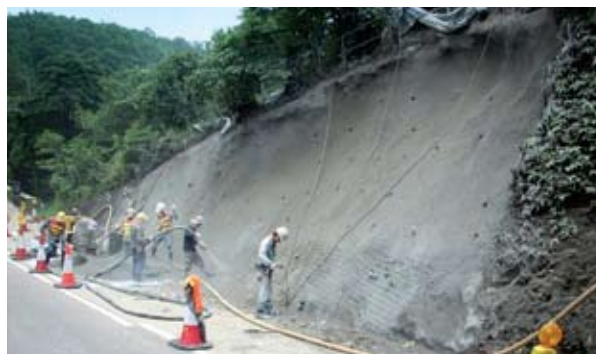
Extraordinary heavy rain on 7 June 2008 resulted in flooding of North Lantau Highway, Hong Kong. Though not part of that highway's maintenance contract, Gammon rapidly deployed to remove the danger and disruption to the public resulting in a letter of appreciation from the Director of Highways.
