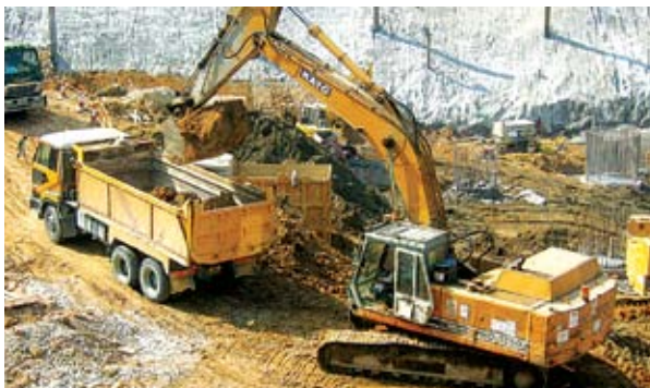
Finding alternatives to Public Fill – Promoting Re-Use In order to make use of construction and demolition (C&D) materials generated by the Tamar Site, Gammon-Hip Hing Joint Venture identified four construction projects where such surplus inert C&D materials was used. Direct reuse of materials reduces transport in and around Hong Kong and reduces burden on Government fill operations.
